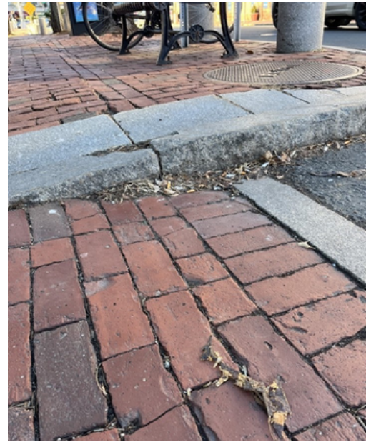
Figures 17 & 18. Observed deficits in brick sidewalks and crosswalks
